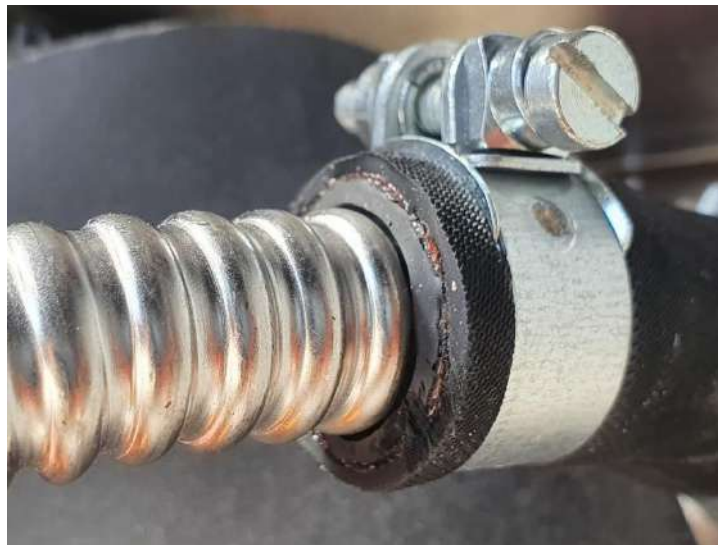
Figure 7: Oil hose on corrugated pipe
