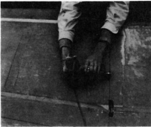
Photo No. 43: Use both hands to control saw. Don't sand before cut.
