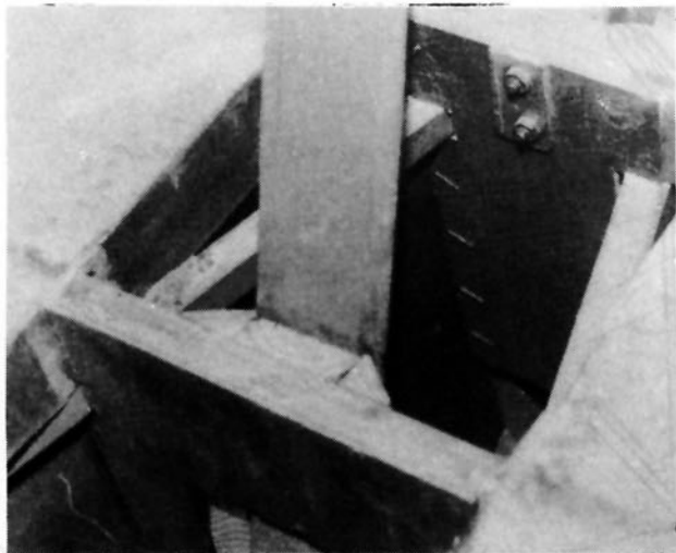
Photo No. 10: Aft plywood web and elevator center hinge plate.
