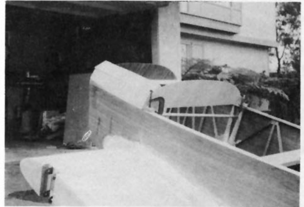
Photo No. 44: Forward deck contour guides. Planking starts.
